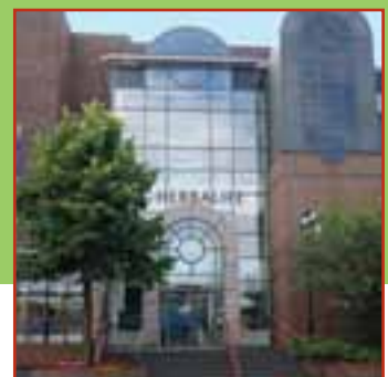
U.K. Distribution Center
