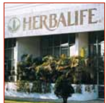
Mexico Distribution Center
